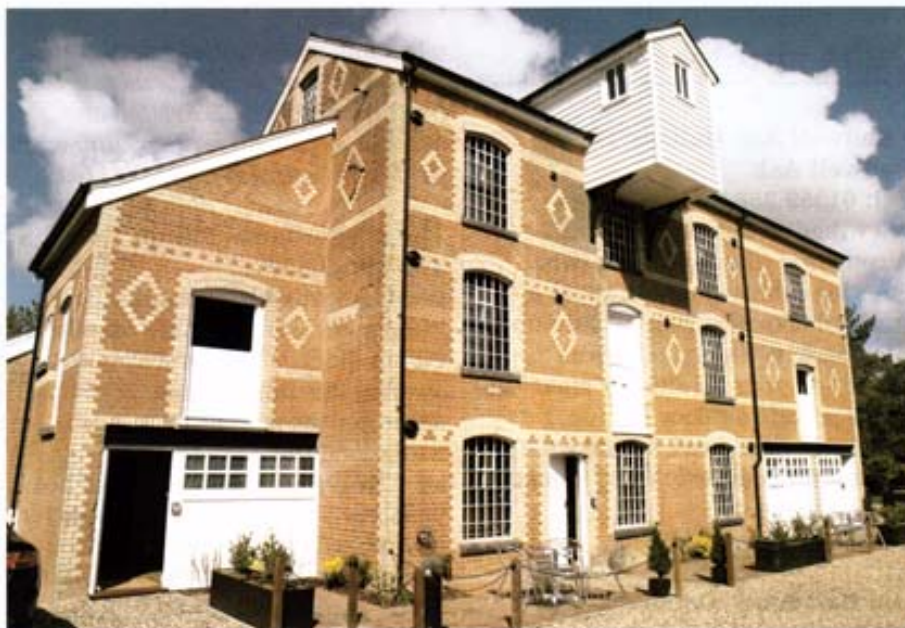
The attractively renovated Swiland Mill, now three self-catering apartments. Left; a view of the stylishly decorated interior
